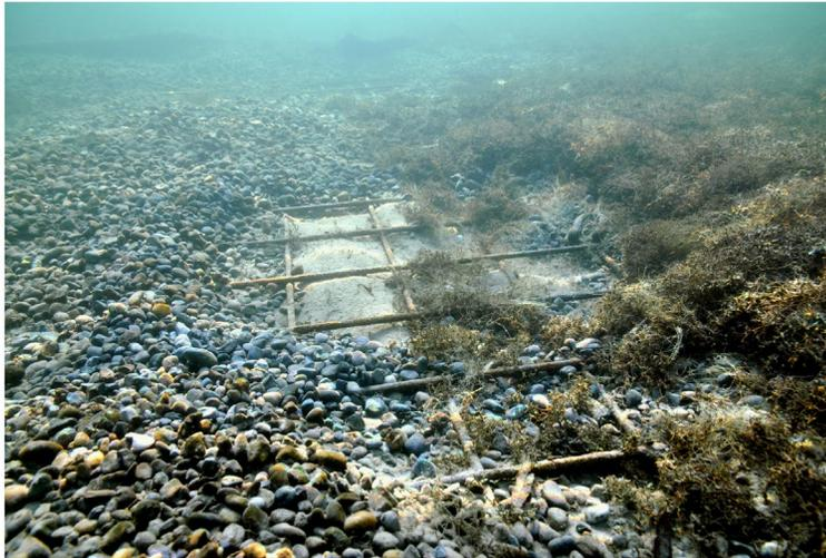
FIGURE 4 Gravel fill at the site Ermatingen-Westerfeld (ERMW) with underlying geo-texile fixed on a reinforcement mat. The exposed geo-texile is the result of grazing activities of mute swans and anchoring of boats.
